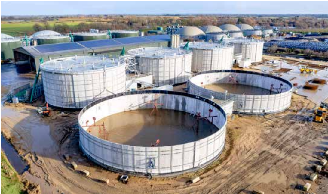
Not exactly small either, like Mepal II, the third plant is designed exclusively to produce biomethane for injection into the grid
