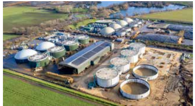
At the time it was built, the Mepal I biogas plant was one of the largest in the world.
