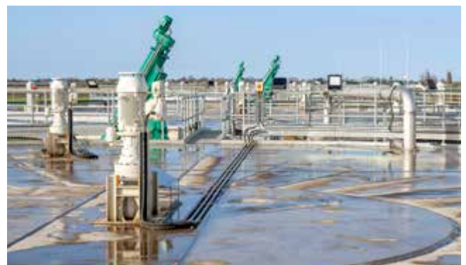
The paddle mixers designed by Agraferm operate at low revolutions, saving energy and reducing wear.
